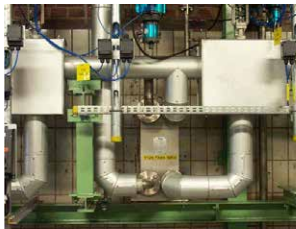
SIGMA WIG ST12 in a heating-cooling circuit for tempering of chemical reactor
